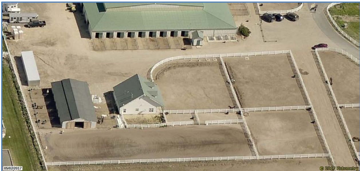
Caretakers quarters and perimeter / internal fencing
